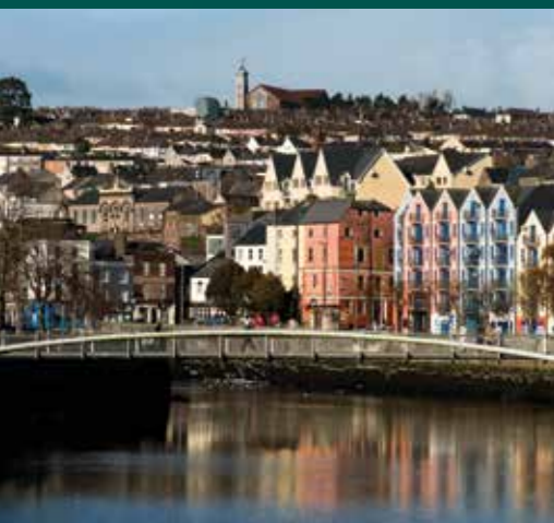
Shandon Bridge over the River Lee, Cork City
